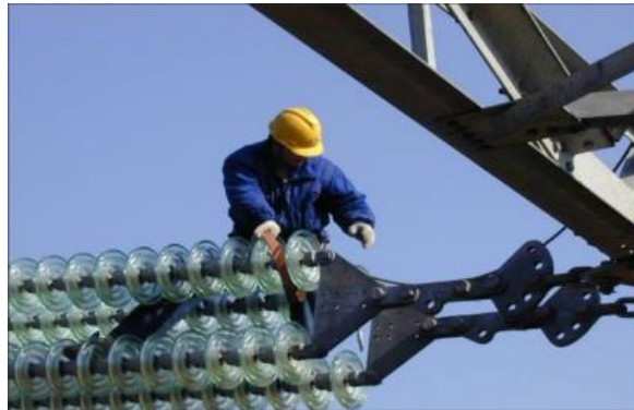
Fig. 5. Hanging insulator string horizontally
