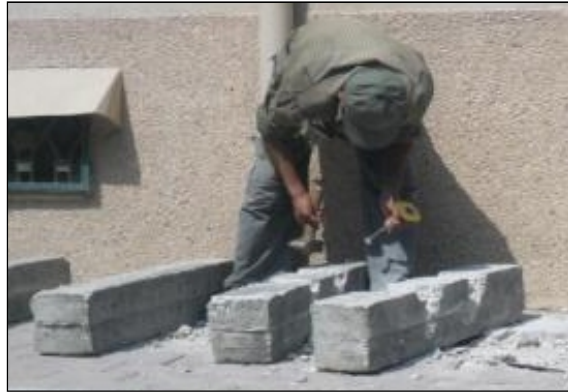
Fig. 3. Cracked beams are V-shaped grooved
