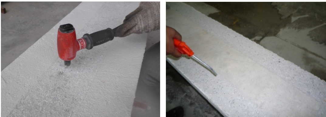
Fig. 1. Preparation of surface
