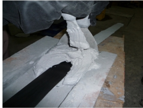
(b) Placing of adhesive on CFRP laminate
