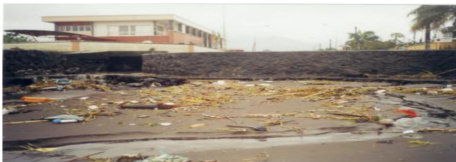
Figure 3. The same road at 'Down Beach' rehabilitated in 2004
