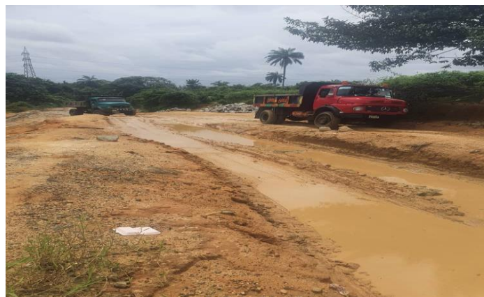
Plate 2. Heavily damaged roads at Choba mining site Source: Researcher's field work (2021).
