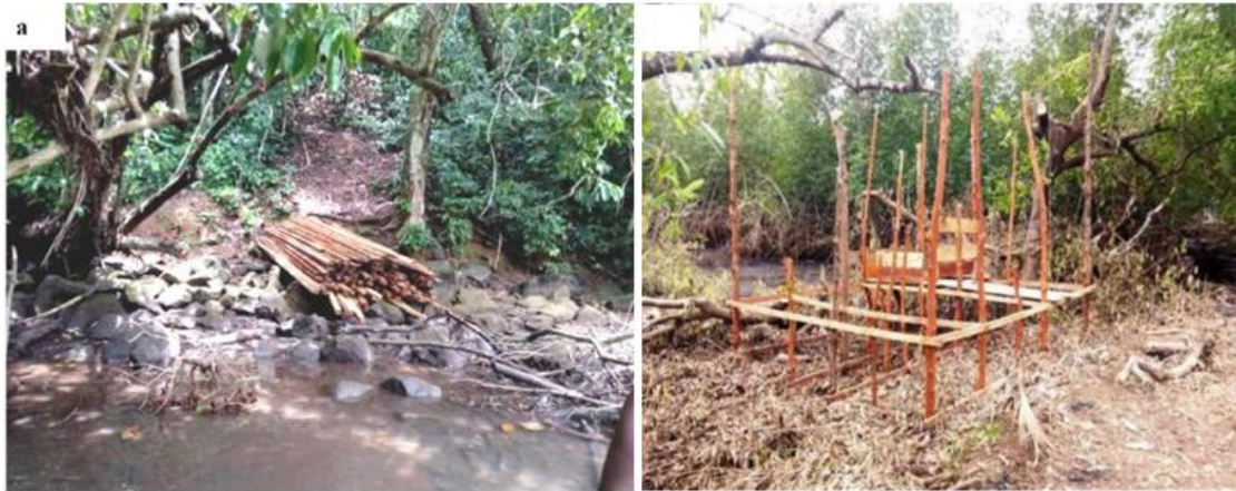
Fig. 6. Building materials (a) Mondoli and (b) Douala Koto beach
