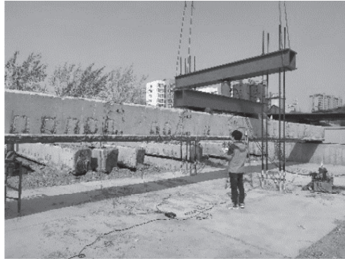
FIGURE 4: The on-site loading situation.
