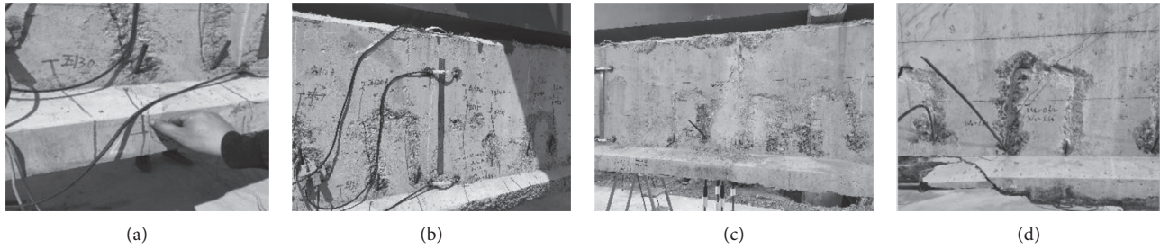
FIGURE 8: The typical failure pattern. (a) No. 2#. (b) No. 3#. (c) No. 4#. (d) No. 5#.
