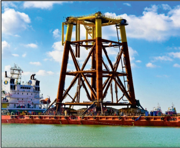
FIGURE 17: Offshore platform jacket.
